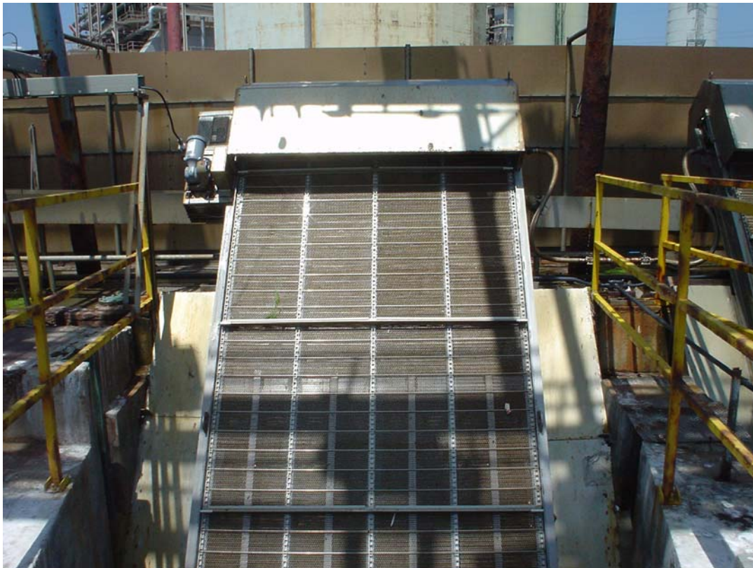
Figure 3.2-3. F.P.I. traveling water screens at the AGS.
